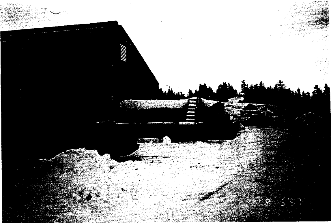
Photo 12 Salt Pond - Building and fuel tank
