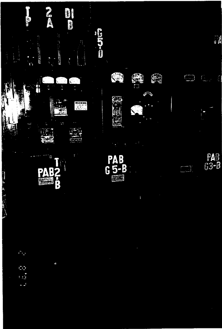
Photo 51 Port-aux-Basques - Outdated switchgear
