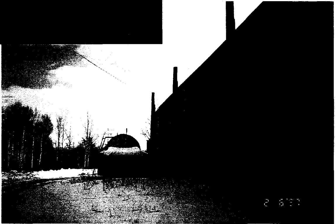
Photo 18 Gander - Exhaust and fuel tank
