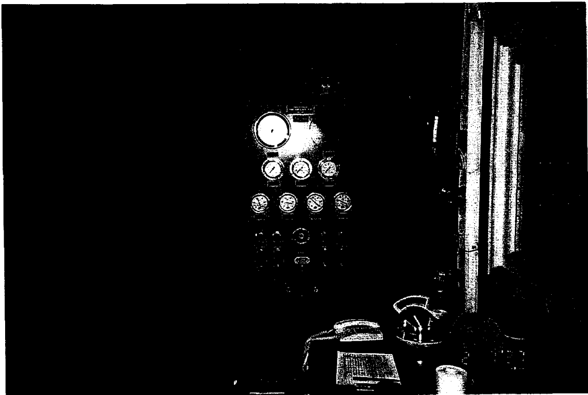
Photo 40 Aguathuna - Engine instrument panel in control room
